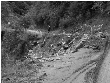
图 7 边坡滑塌 Fig. 7 Slope landslide
